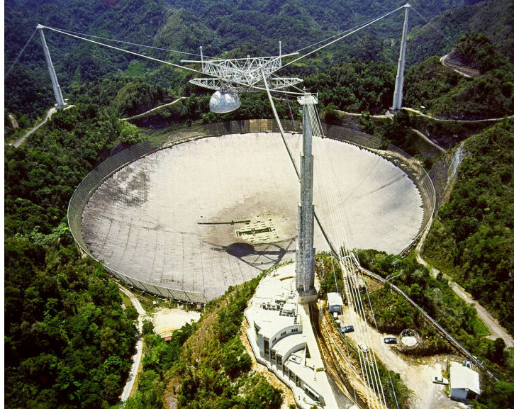
Figure 16: The Arecibo Radio Telescope, at Arecibo, Puerto Rico. At 1000 feet (305 m) across, it is the second largest dish antenna in the world. The dish, built into a bowl in the landscape, focuses radio waves from the sky on the feed antenna suspended above it on cables. Since the dish itself can't move, the telescope is steered to point at different regions of the sky by moving the feed antenna (dome) along the curving metal track. It is used in three major areas of research: radio astronomy, atmospheric science, and radar astronomy. Scientists who want to use the observatory submit proposals that are evaluated by an independent scientific board. The observatory has appeared in film and television productions, gaining more recognition in 1999 when it began to collect data for the SETI@home project. Picture from https://commons.wikimedia.org/w/index.php?curid=16005203
